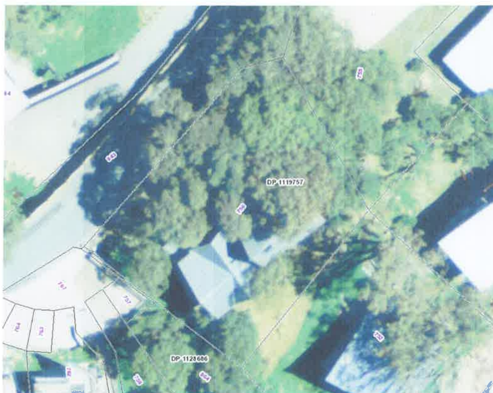
Figure 6: Aerial view of Athol Lodge showing the roof.
