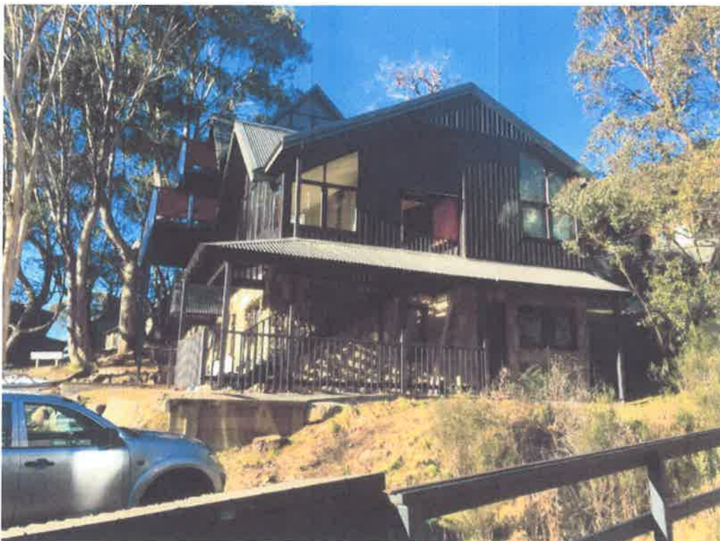
Figure 12: Western facade of Athol Lodge. Source: Elizabeth Pugh Building Design
