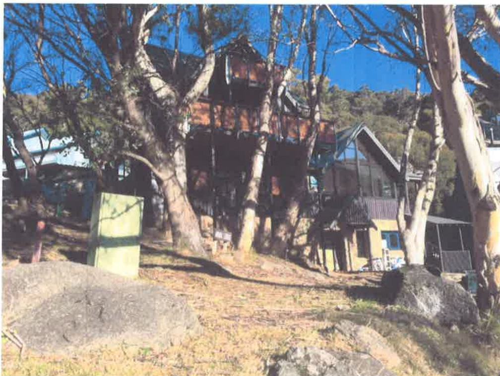
Figure 10: Front facade of Athol Lodge Source: Elizabeth Pugh Building Design
