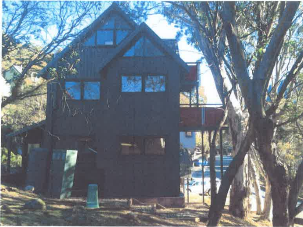
Figure 9: Front facade of Athol Lodge. Source: Elizabeth Pugh Building Design
